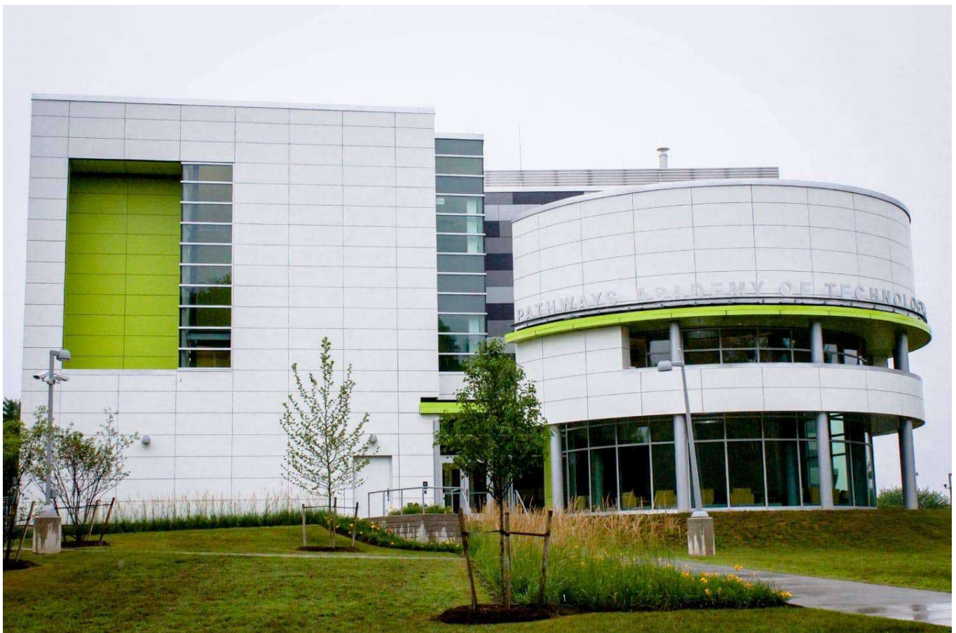
Pathways Academy of Technology & Design at Goodwin College | Photo Credit Roof Tech Sales
