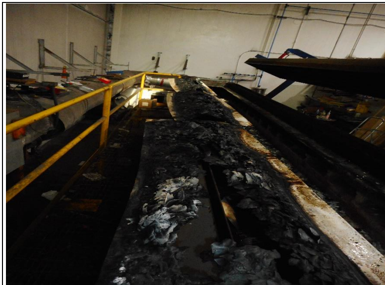
Photo No. 2 Post Test
