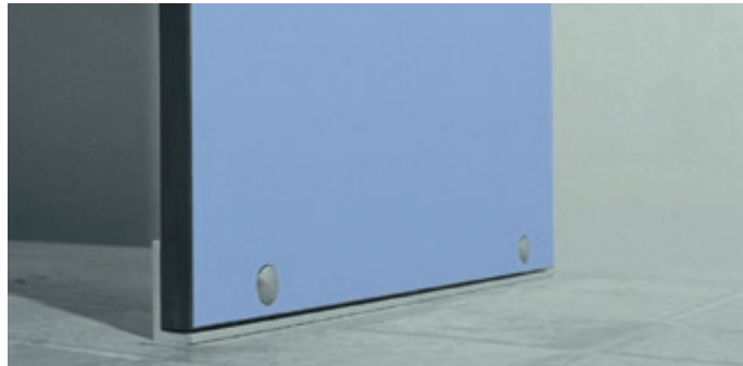
FLOOR CONNECTION WITH L-PROFILE
