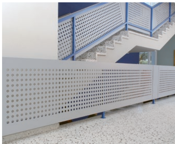
STAIR RAILING - HOLE MILLING
