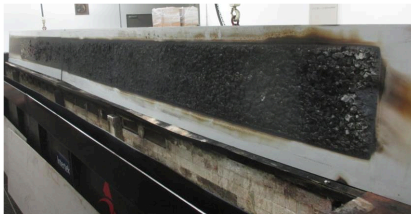
Photo No. 4 Exposed Surface of the Test Specimen (Post-test)
